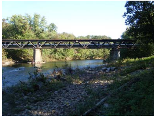
Looking At: Downstream Face
