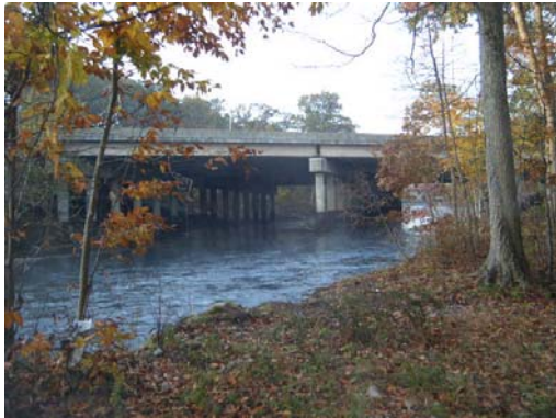
Looking At: Upstream Face
