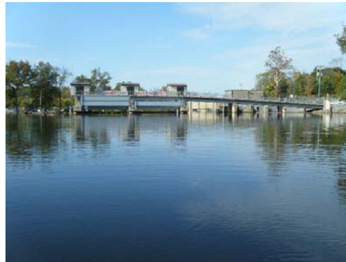
Looking At: Downstream Channel
