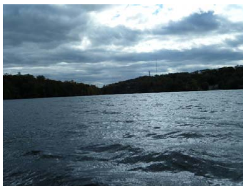
Looking At: Downstream Channel
