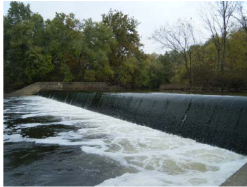
Looking At: Downstream Face
