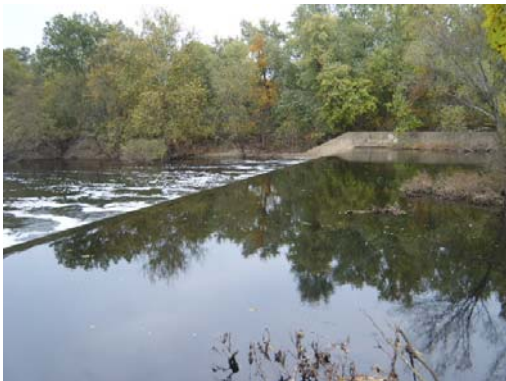
Looking At: Upstream Face
