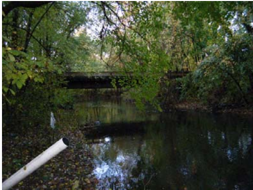
Looking At: Upstream Face
