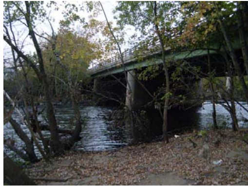
Looking At: Downstream Face
