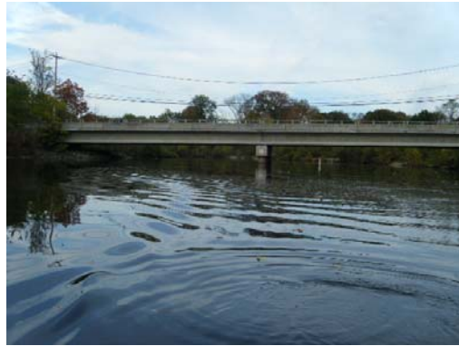
Looking At: Downstream Face
