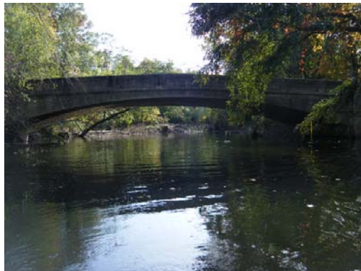
Looking At: Upstream Face
