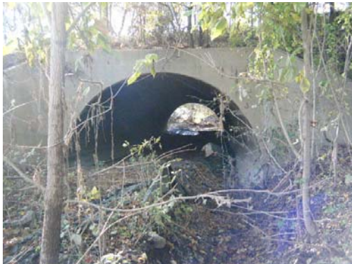
Looking At: UPSTREAM FACE
