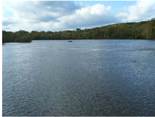
Looking At: Downstream Face
