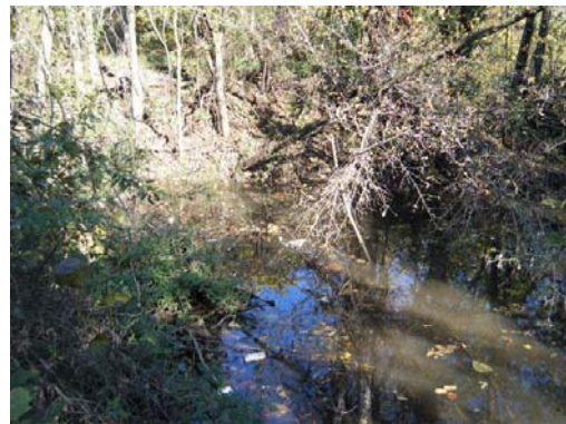
Looking At: DOWNSTREAM FACE
