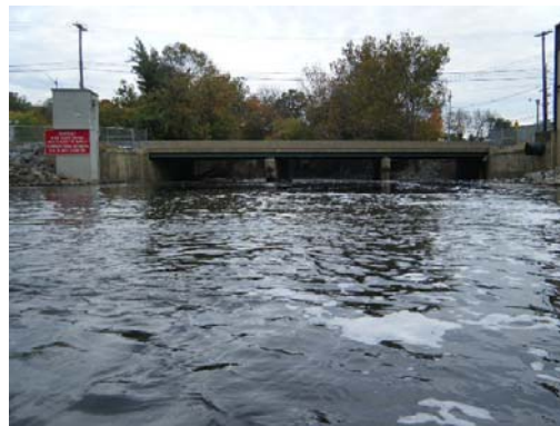
Looking At: Downstream Channel
