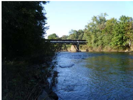
Looking At: Upstream Face
