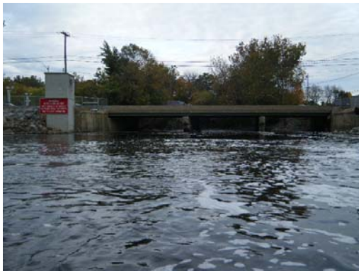
Looking At: Upstream Face
