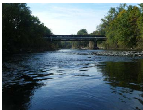
Looking At: Downstream Channel
