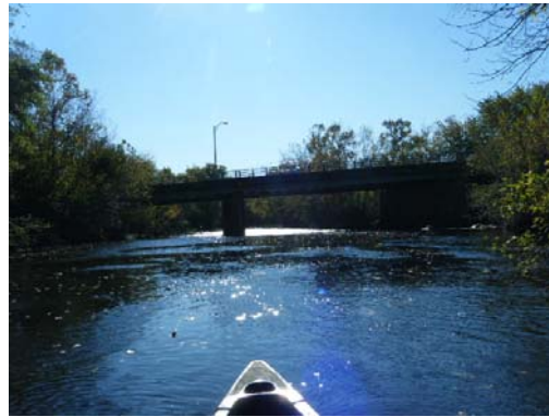
Looking At: Downstream Channel
