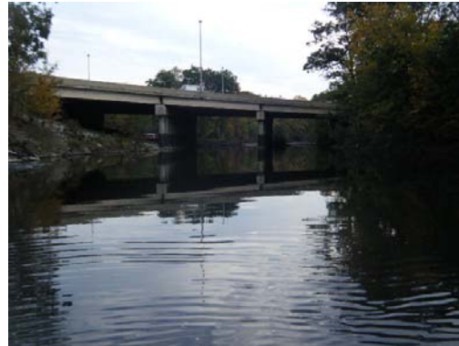
Looking At: Downstream Face
