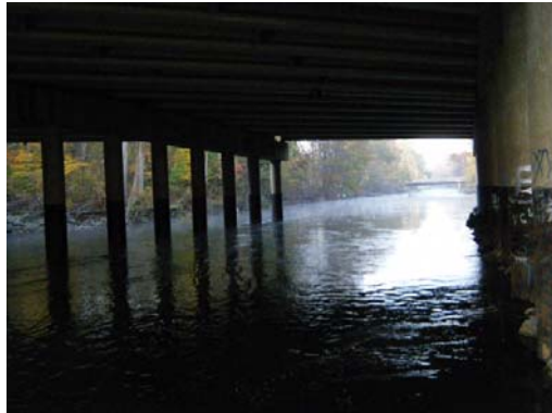
Looking At: Downstream Channel
