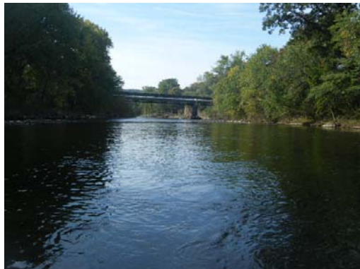
Looking At: Upstream Face
