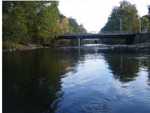
Looking At: Downstream Face
