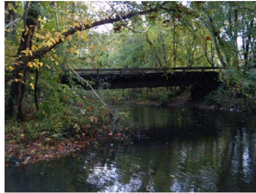
Looking At: Downstream Face
