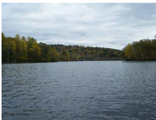
Looking At: Downstream Channel
