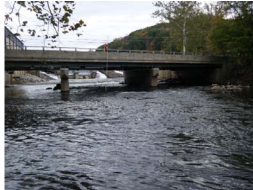
Looking At: Downstream Face
