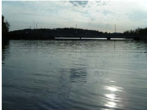
Looking At: UPSTREAM FACE
