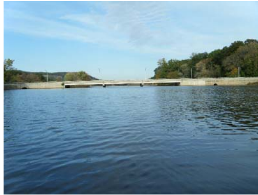
Looking At: DOWNSTREAM FACE
