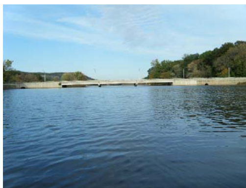
Looking At: Downstream Channel
