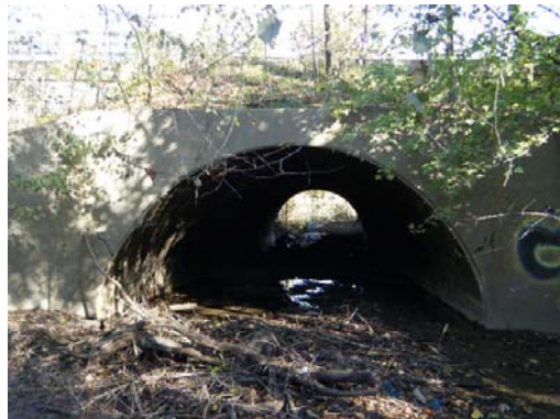
Looking At: DOWNSTREAM FACE
