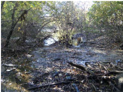
Looking At: DOWNSTREAM CHANNEL
