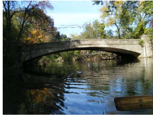
Looking At: Downstream Face
