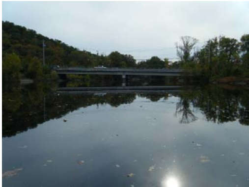
Looking At: Upstream Face
